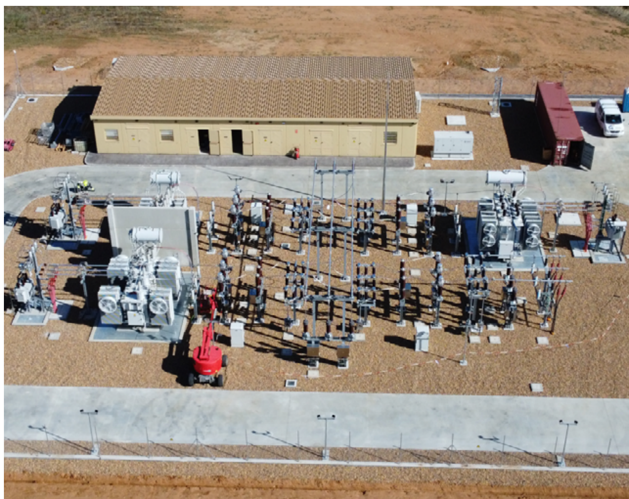
Digital substation Majuelo 66/30 kV
